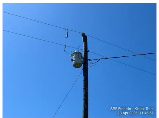
Photograph 13: View of a pole-mounted transformer located on the northern portion of the Subject Property along Allen Road. A non-PCB sticker was not observed, and no stains or leaks were noted.
